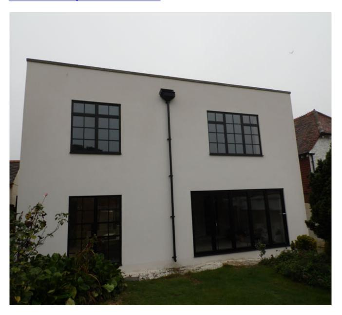
As the design was to give the rear of the property an art deco feel, high specification black aluminium windows and doors were installed along with a striking brilliant white render to the external walls and the works were carried out to a very high standard in order to meet the client's requirements
